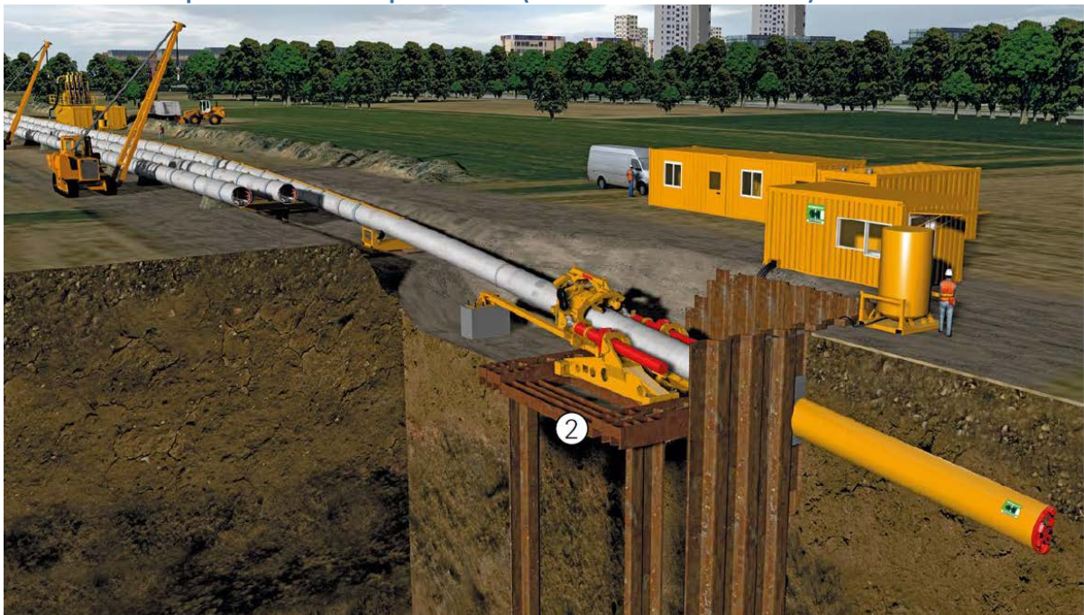
Plate 3: Typical Direct Pipe® onshore arrangement
